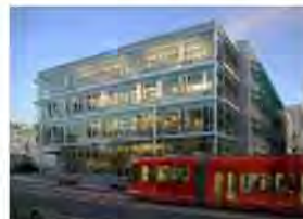
Seattle's Terry Thomas Building, at dusk
